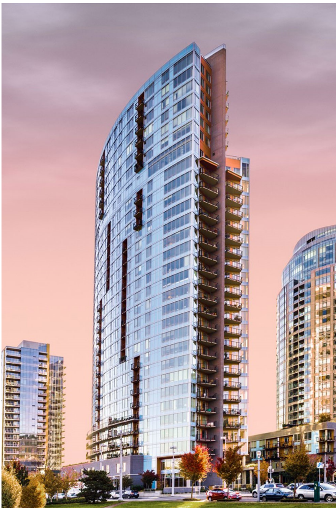
OPACI-COAT-300® Project: Mirabella, Portland, OR, USA 1 st LEED Platinum Continuing Care Retirement Community
